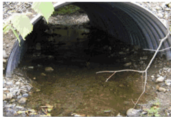
Pipe arch used for stream crossing
