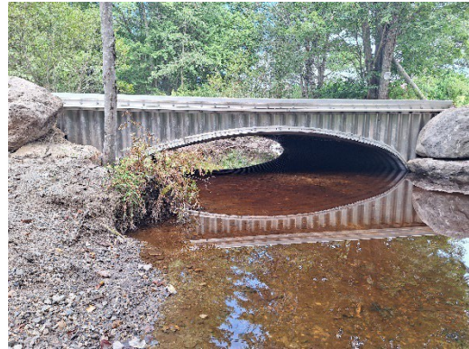
Haskell Brook tributary to Pleasant River (Windham) NPS Project #20210005. Photo on the left shows aftermath of road washout in the Spring 2023, and the open bottom arch crossing installed using CWA section 319 funds in the Fall of 2023. The project prevents 51.29 tons of sediment and 43.6 lbs of phosphorus from entering Haskell Brook each year. Note stream bed restoration efforts as well as crossing stabilization.
