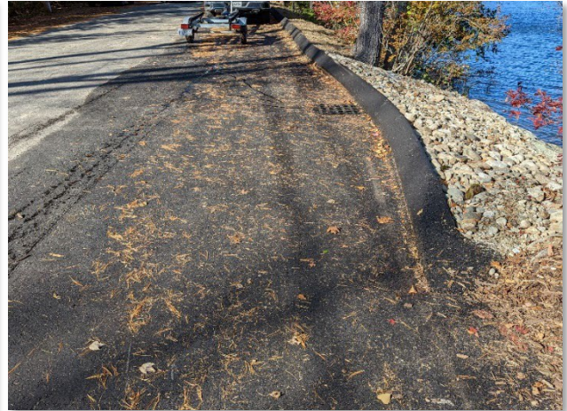
Curbing and catch basin installed at boat launch to stabilize soil and redirect runoff away from the pond
